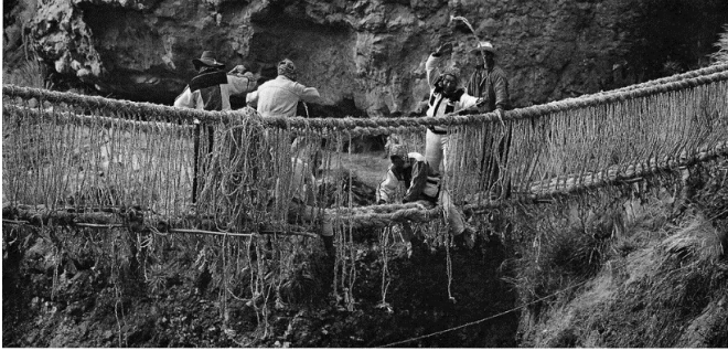
Men from the Quehue district working together to rebuild the Q'eswachaka Bridge using braided, dried grass.
